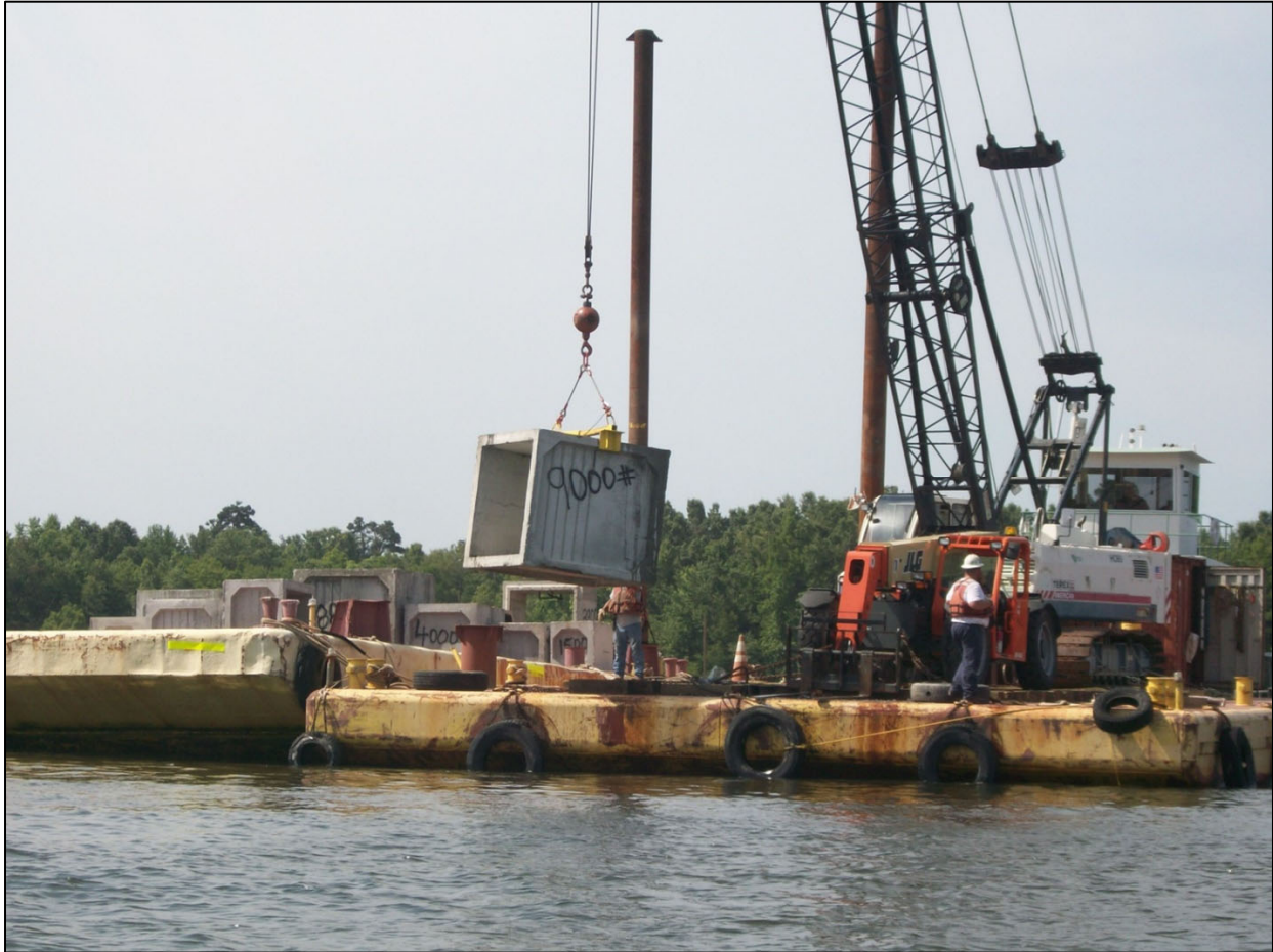
Figure 4.2 – Santee Cooper Barge & Crane Installing Fish Attractors in 2023
